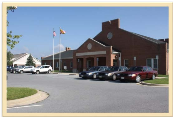
MARYLAND STATE POLICE BUILDING LOCATED AT 1100 BALTIMORE BLVD. WESTMINSTER, MARYLAND 21157
